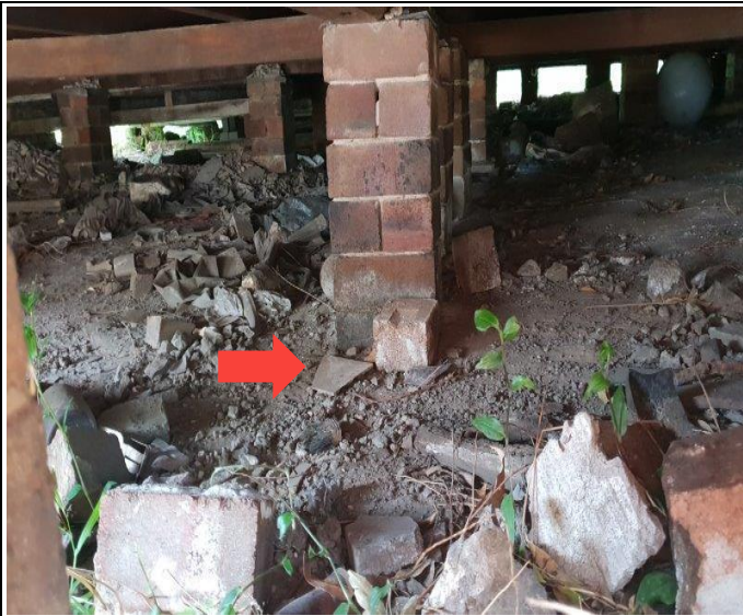
Photo 1: 59 Cowper Street, western aspect to subfloor, fibre cement material observed.
