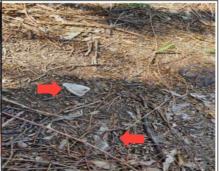
Photo 2: 59 Cowper Street, north western aspect, asbestos-containing fibre cement fragments identified on ground surface.
