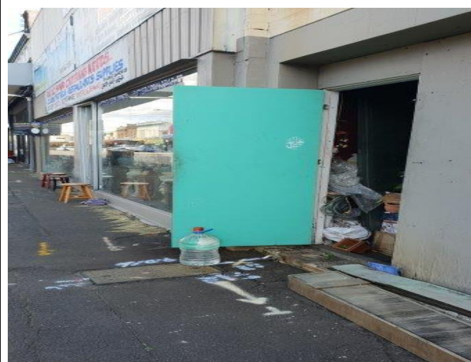
Photo 23: 32-34 Good Street, Shop front façade, lead containing grey paint (WSP-104450).
