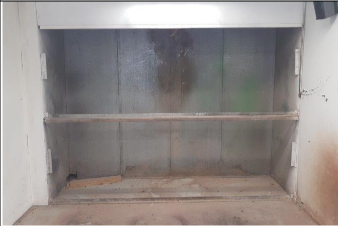
Photo 27: 138 Parramatta Road, spray booth, lead containing white paint (WSP-104443).
