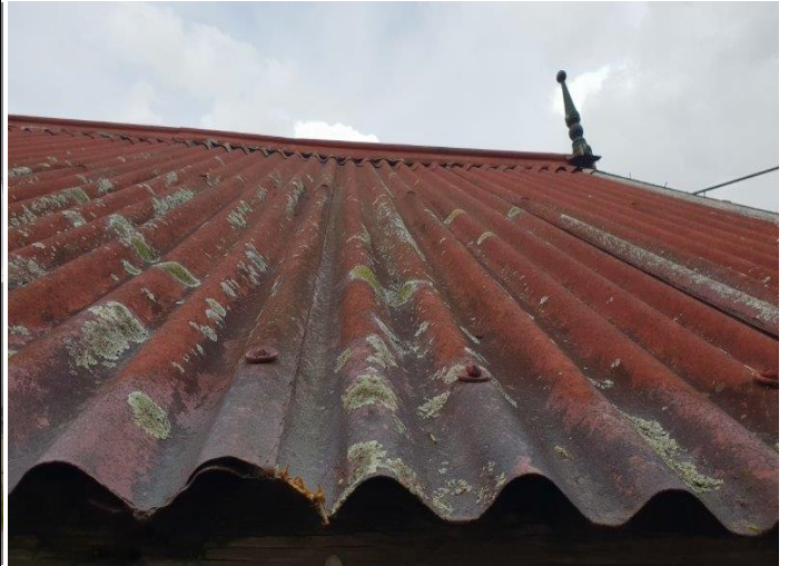
Photo 20: 59 Cowper Street, Dwelling – Exterior, Steel roofing, lead containing red paint (WSP-104430).
