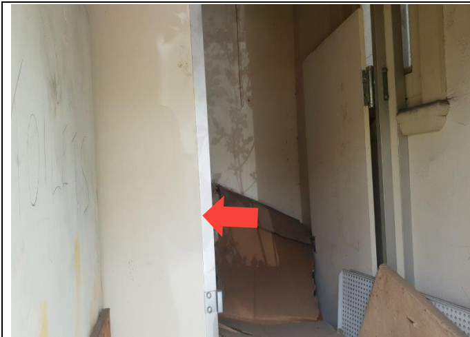
Photo 13: 38 Good Street, Western Elevation - Male Toilets partition walls, asbestos-containing fibre cement Sheetting.
