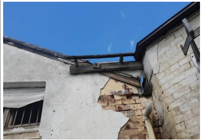
Photo 22: 28-30 Good Street, Bricked walls beneath cement render façade, lead containing white paint (WSP-104452).
